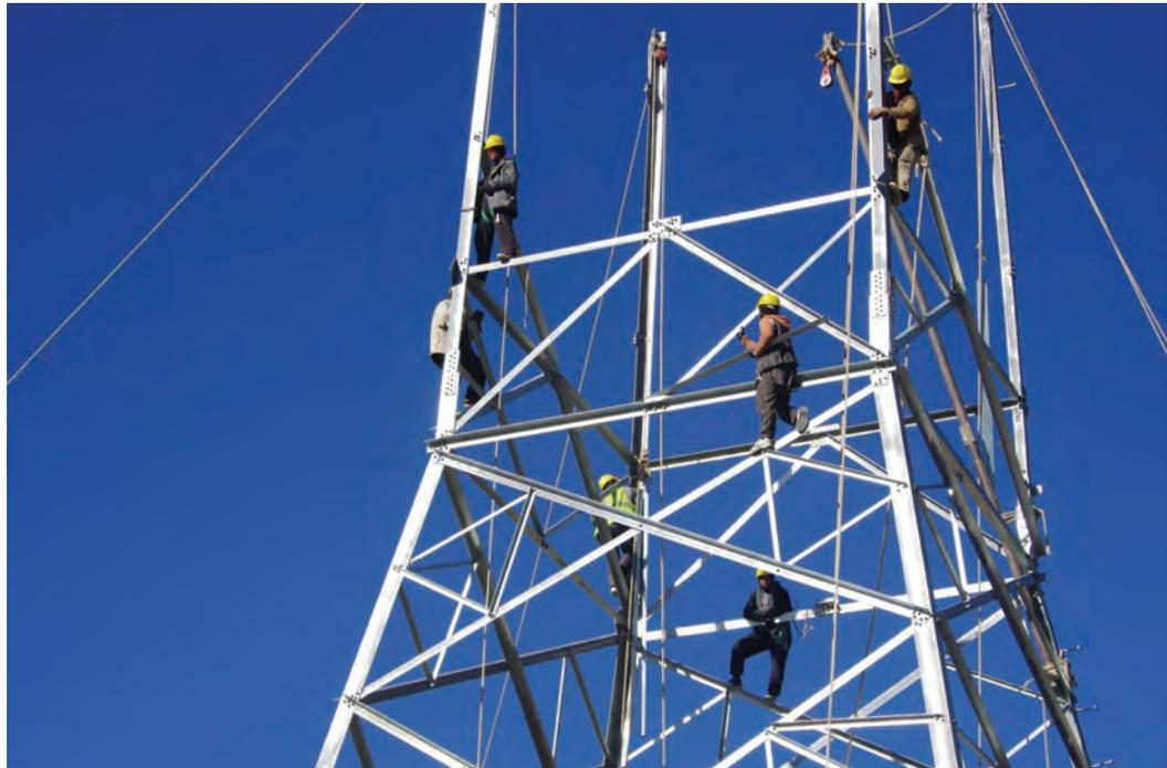
Workers assemble a transmission line tower. The Engineering Support Program provided construction management services and quality assurance for many of USAID's power-infrastructure projects. (USAID photo)
